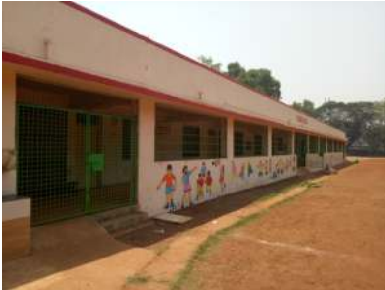
← School Building and Roof area
