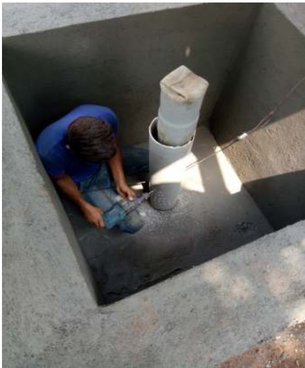
Recharge Pit Construction
